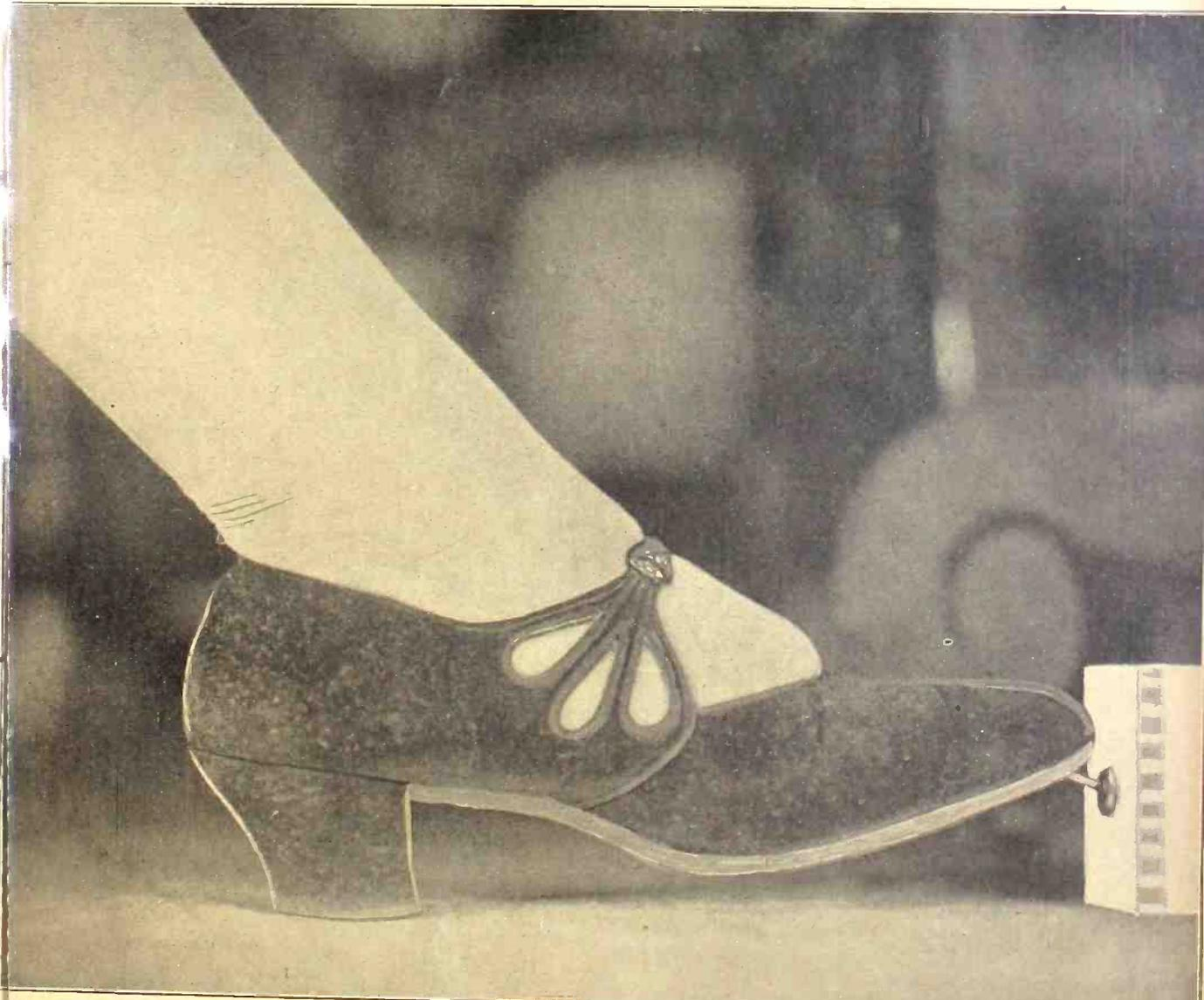
THE UTMOST IN CONVENIENCE!—A switch in a box, secured to the floor, under the table permits Milady to turn the set on or off with no more movement or effort than summoning the maid. (Hayden)
