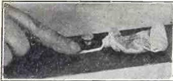
**TOOTHPASTE** may be used to plug up a small hole in a panel or socket shelf. After it hardens, blacken it with shellac.
