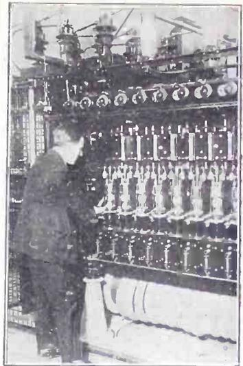
A GENERAL view of the power unit in the new and world's most powerful commercial wireless station, at Hillmorton, England, near Rugby. The station opened on New Year's day. The wavelength is 6,000 meters, power 100 kw. (International Newsreel)
