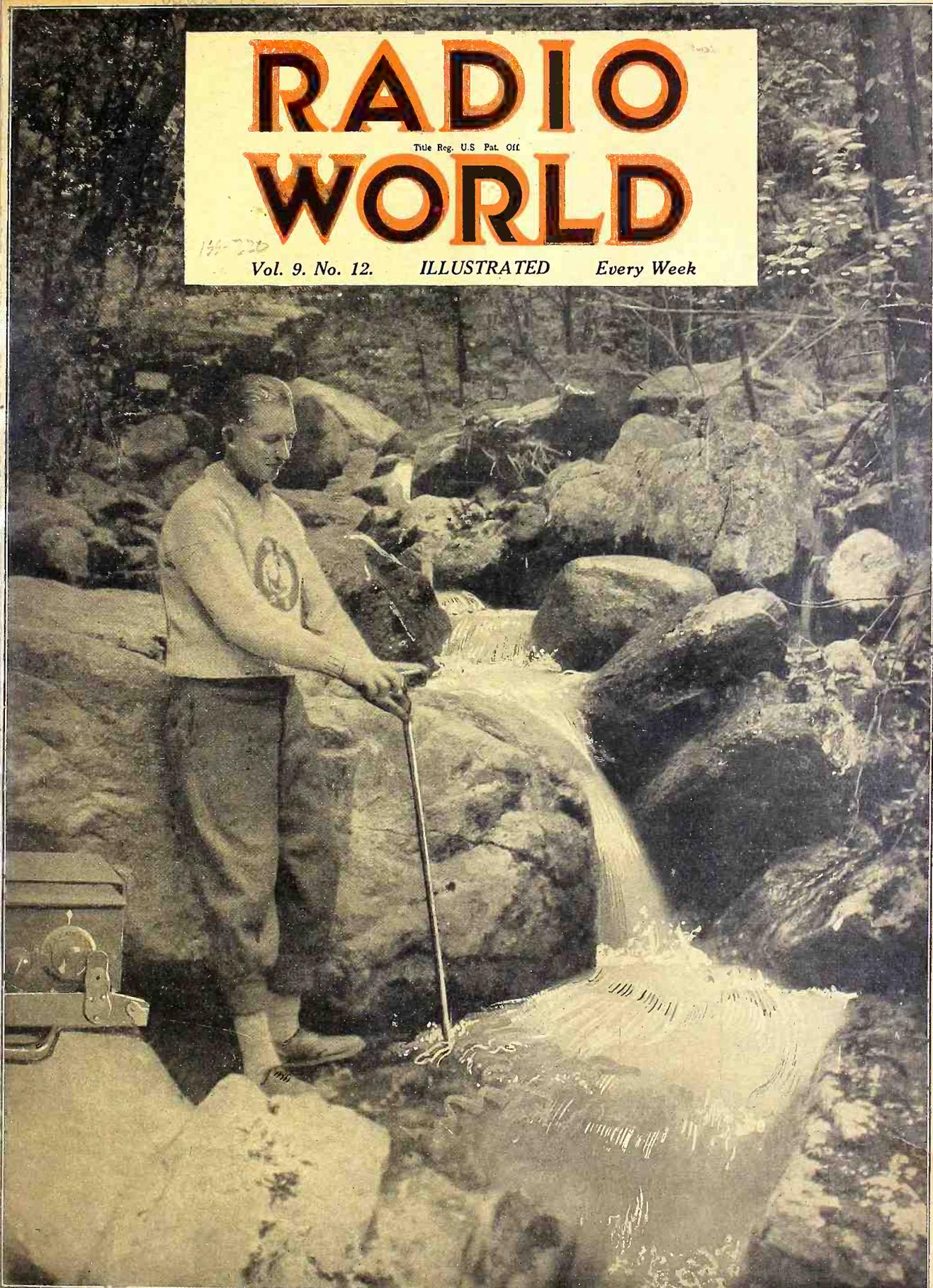
AN IRON ROD in a stream bed makes a good ground. See Pages 16 and 17.
