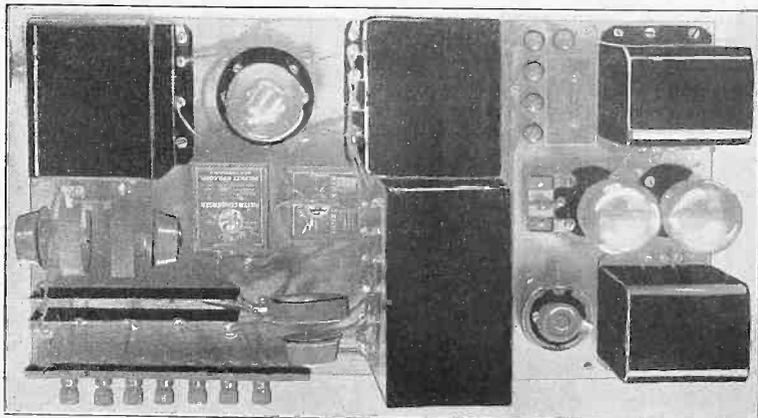
LAYOUT FOR THE G. R. PUSH-PULL AMPLIFIER TYPE 441, AT RIGHT, WHEN USED WITH A POWER AMPLIFIER, AT LEFT, USING THE GENERAL RADIO TYPE 365 RECTIFIER TRANSFORMER AND TYPE 366 CHOKE COIL, IN CONJUNCTION WITH THE Q. R. S. 85 MIL RECTIFIER TUBE, POLYMET HI-VOLT CONDENSERS AND CENTRALAB VARIABLE RESISTORS.
