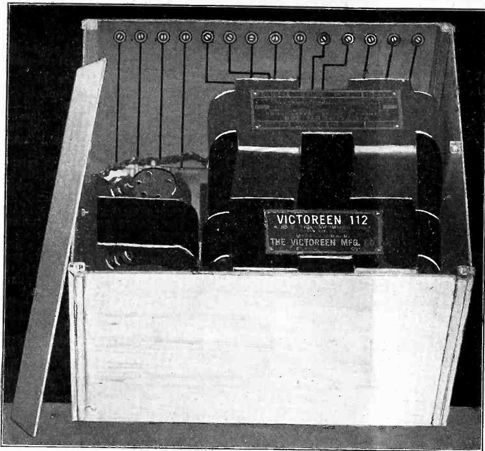
AN ANGULAR SQUINT AT THE AC FILAMENT SUPPLY AND AUDIO AMPLIFIER SHOWS THE TOP AND THE PARTITION OF THE SHIELD REMOVED. PLACEMENT OF THE 112 TWO-STAGE AUDIO AMPLIFIER AS SHOWN KEEPS THE GRID LEADS AWAY FROM THE FILAMENT TRANSFORMER. THE BINDING POSTS TOWARD THE LEFT ARE FOR FILAMENT SUPPLY OUTPUT, TO SERVE EXTERNAL TUBES. THOSE TO THE RIGHT ARE INPUTS FROM A B POWER DEVICE.
