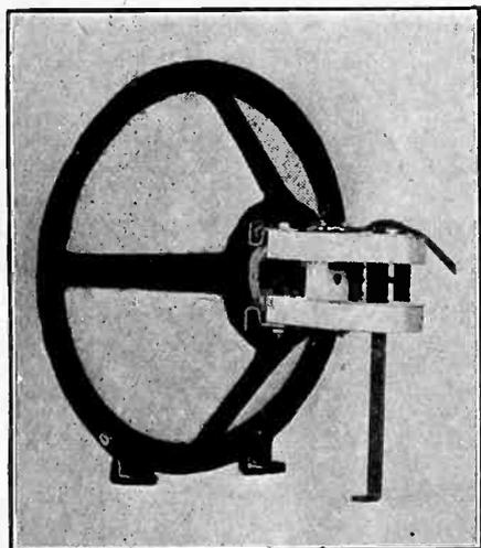
Absolutely the best tone quality, with amazing sensitivity, is assured when you use the Inductor Speaker on a fine audio amplifier. The chassis is sold completely erected with a supporting brace. The unit, cone spider and ring, are sturdily put together. Use a baffle board or box of your own choice. Baffle instruction sheet in each carton.
