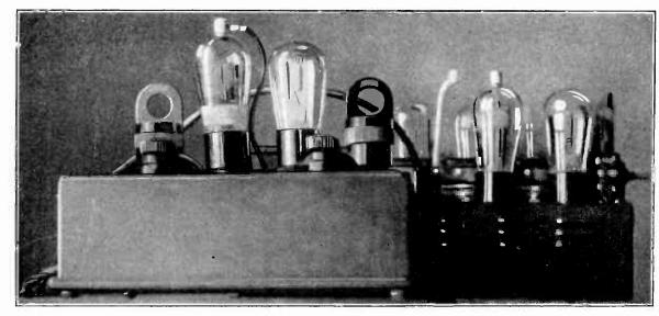
THE ADAPTER HOOKED UP TO A TWO-STAGE SCREEN GRID RF RE-CEIVER, THE 6-TUBE NJ-30 OF THE JACKSON LABORATOR-IES, ON WHICH IT WORKED FAIRLY WELL. THE SIXTH TUBE IS THE
