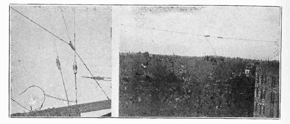
Haywire roof aerials of an apartment house, at left. A doublet antenna strung in the clear, at right.
