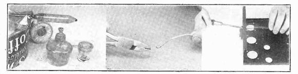
Can't read the brand of coffee on the label, but can is upside down, tin cover cut to remove coffee (just as important as anything else), and elevated resting place provided for soldering iron that needs alcohol lamp or pepper pot soup to become useful. Special pliers make neat lug end on wire. Socket wrench spares fingers for tightening in cramped places.
