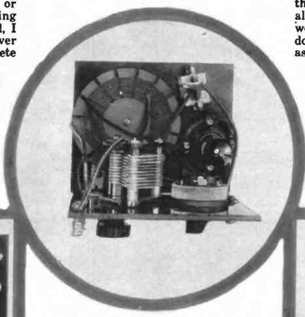
Above is a view looking directly down upon the baseboard showing how the spiderweb coils are placed so that part of them come underneath the variable condenser. To the left and right are rear views showing the placing of the various instruments on both panel and baseboard
