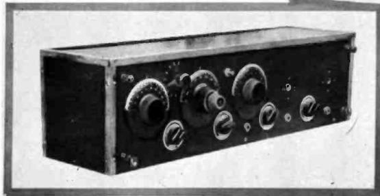
the market. I refer to the Calvert knock-down cabinet. I am showing it in the illustration in the form in which it came to us, all taken apart and folded up neatly in tissue paper in a box, and I am also showing it put together with a screw driver ready to slip the set in.
