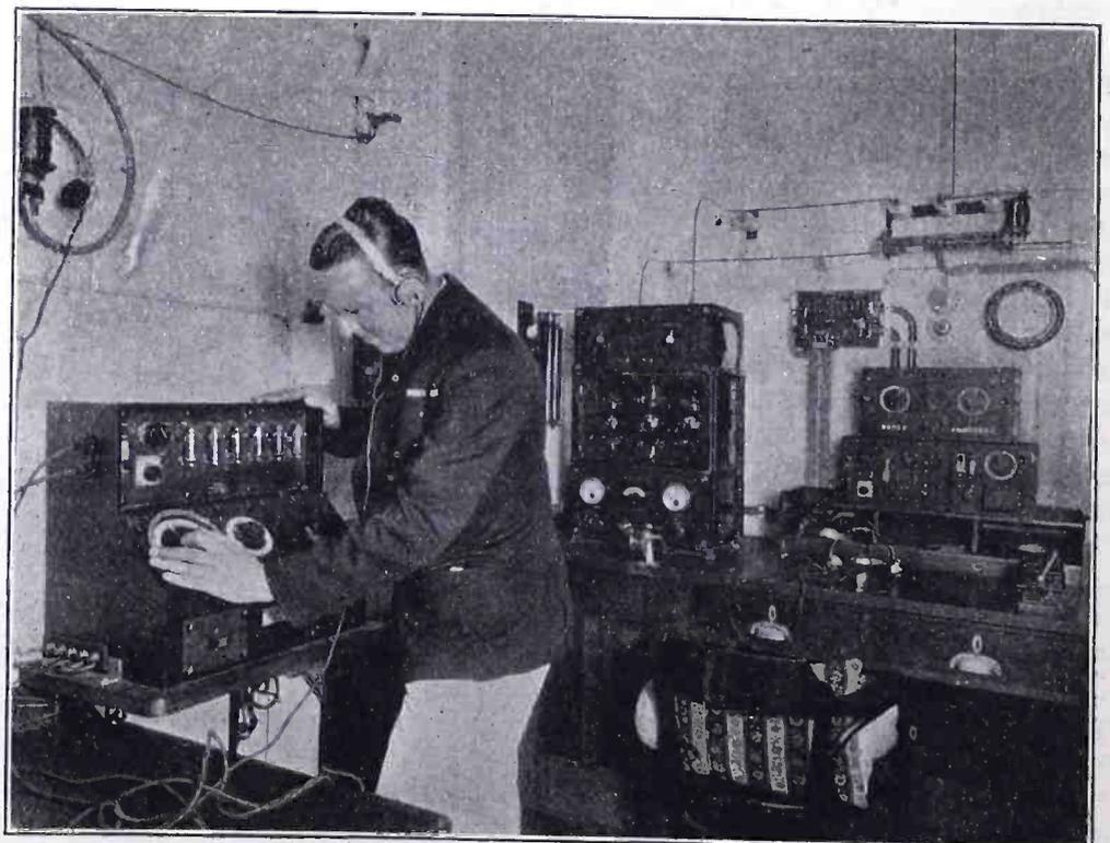
$1\frac{1}{2}$  K. W. Tube Transmitter on S. S. "Majestic" showing Operator Brunt using "D. F." Radio Compass
