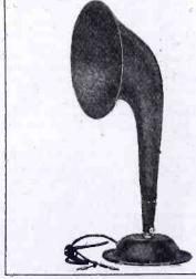
The Bristol "Baby Audiophone" is a model with fiber horn as illustrated. It is attractively finished in dull gold bronze. It gives a natural tone without mechanical distortion with sufficient volume to be heard in a large room.
