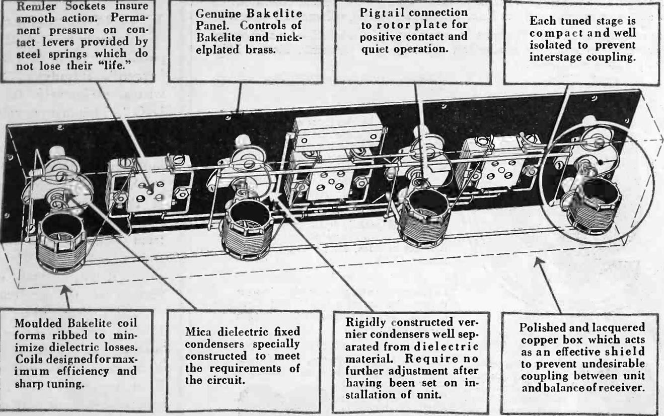
Remler Sockets insure smooth action. Permanent pressure on contact levers provided by steel springs which do not lose their "life."
