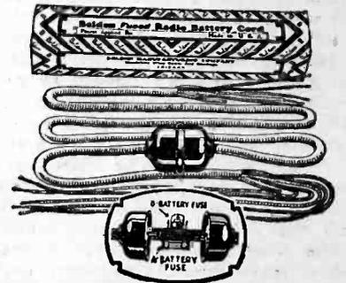
on the cord and are protected by a bakelite shield which may be opened for inspection or replacement. This cord protects tubes and batteries against accidental over-voltage and does away with the unsightly mass of wires frequently used to connect the batteries to a set.
