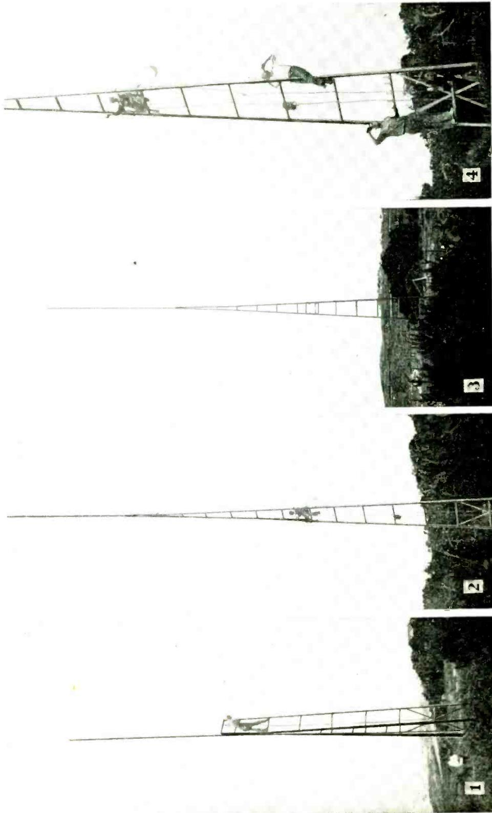
Figure 1 shows the bottom section guyed in place and the top section raised on the ground. Figure 2 shows the top section being bolted into place. Figure 3 shows the completed job, and Figure 4 the "steam beer" method of pole raising.
