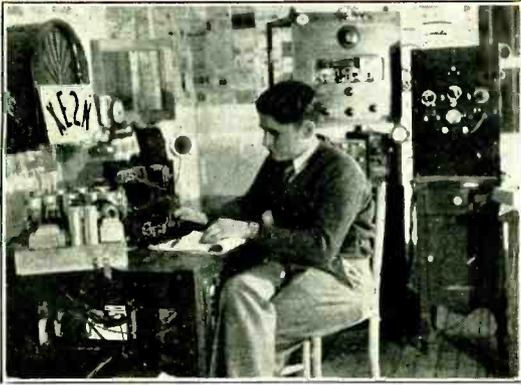
Juan Lobo, XE2N, Monterrey, N. L. The unit on the extreme right is the all-band exciter. Just behind the key is the modulator, built during the first four hours of the phone dx contest.
