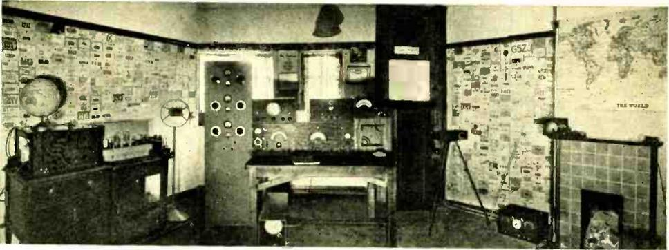
**G5ZJ** at Letchworth, England, operated by Kenneth Jowers primarily on 10- and 20-meter phone. Over 90 countries and 27 zones have been worked on phone. From left to right can be seen the cathode ray equipment, speech amplifier, low-power emergency transmitter, main transmitter using a pair of 100th's, u.h.f. receiver preselector, main receiver, mixer panel, 5-meter transceiver, and three-band exciter having 12 crystal frequencies.
