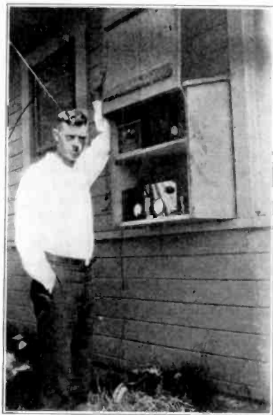
Outside Transmitter at 6BDR
