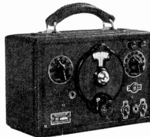
RCA Test Oscillator, Type TMV-97-C, range 90 to 25,000 kc., covering all r-f and i-f alignment points. For use separately or with Oscillograph. \$34.50.
