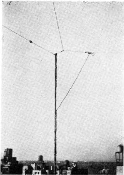
Fig. 2. Typical iron-pipe mast for master antenna system.
