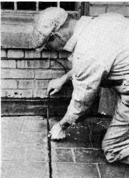
veniently located on a parapet or side wall. The ground connection is made to the roof flashing or to a standpipe known to be properly grounded.
