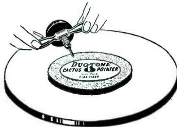
needle sharpener which utilizes the turntable of the phonograph motor for drive power.
