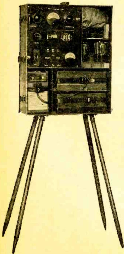
Fig. 13, at the left, shows a Lorenz 2-watt, short-wave portable transmitter. In this apparatus, which is shown here with demountable legs, the transmitter and the sources of power are all combined into a single container. The ground radiation of this transmitter permits telegraphy up to about eighteen miles. After bridging first dead zone, they can be heard by space radiation, up to several hundred miles.
