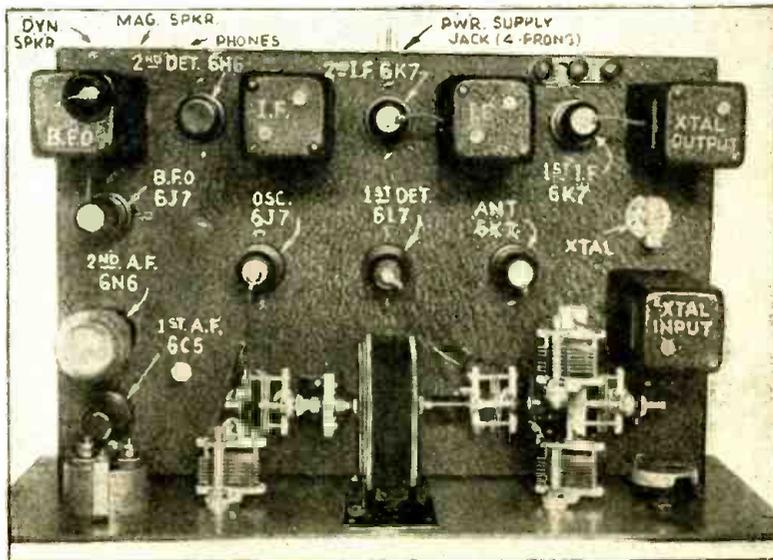
Fans and Hams alike will be pleased with this very flexible superhet design. It may be built with as low as seven tubes if the beat oscillator and crystal filter are dispensed with.
