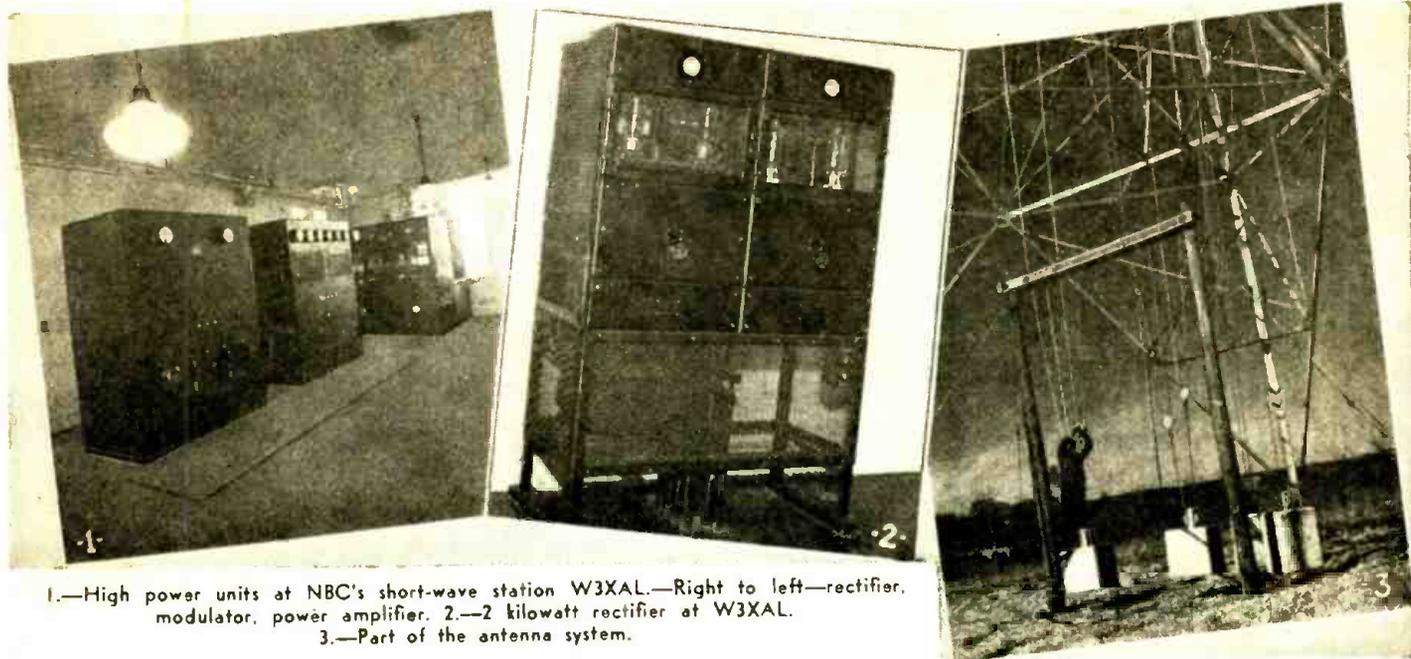
1.—High power units at NBC's short-wave station W3XAL.—Right to left—rectifier, modulator, power amplifier. 2.—2 kilowatt rectifier at W3XAL. 3.—Part of the antenna system.
