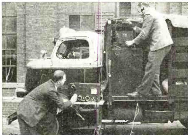
testing the radio equipment on one of the trucks which the expedition includes. A trailer and a cruising sedan will also be employed. The system, powered by standard car batteries, is similar to that used by many police departments. Antennas, ranging from the standard fishpole type to a 128-foot flat-top, are being provided.
