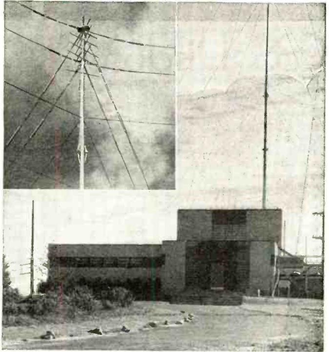
Photo at left shows Harry Whitmore at the transmitter panel of WIXOJ, frequency modulated station at Paxton, Mass. Photos at right show transmitter building at Paxton; 50 kw. equipment under construction. Insert shows transmitter antenna mast, with 4 bay turnstile aerials and vertical aerial on the peak.
