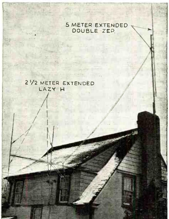
Left—Close-up view of the 2½ meter transmitter. Right—The antennas used at Station W2DKJ for 2½ meter operation.
