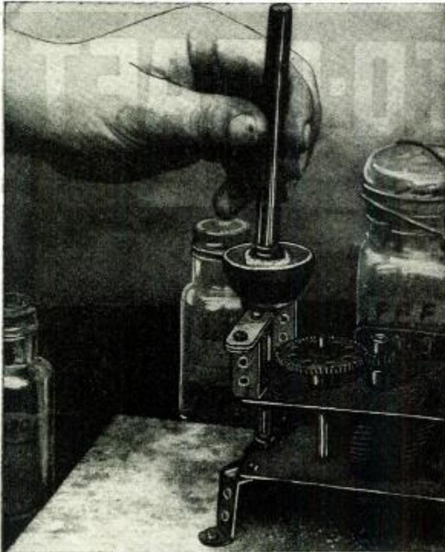
Grinding a lens on a phono-motor driven lap.
