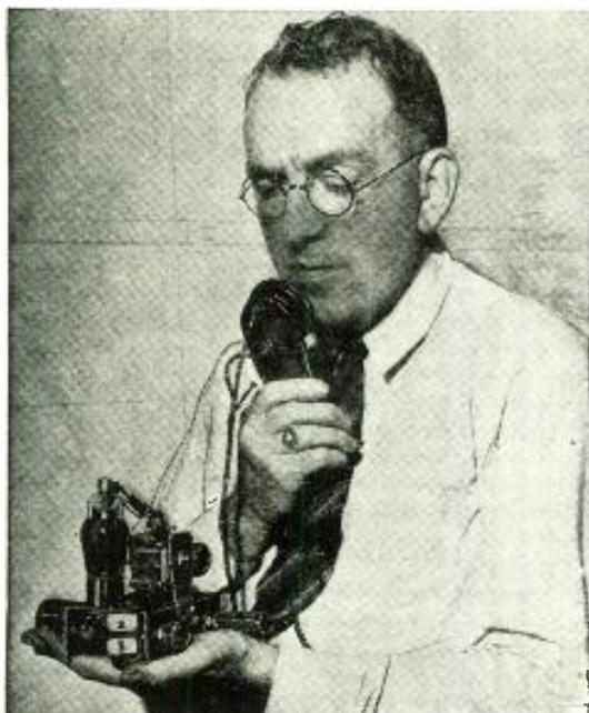
The flea-power transceiver in operation; it plugs into any lamp socket for its power supply.
