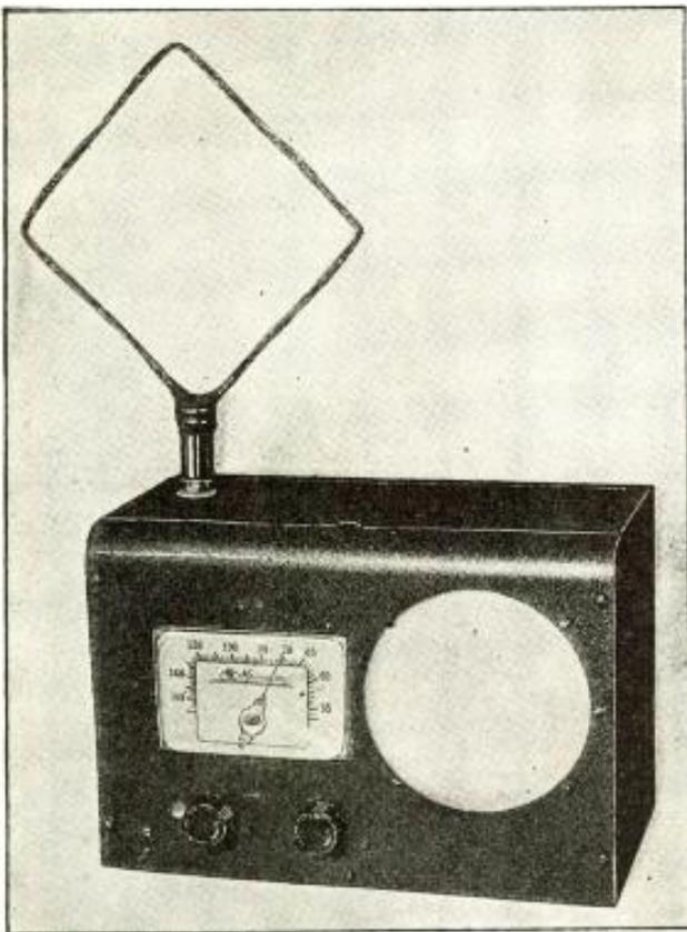
The loop antenna on this portable is removable. It was designed to plug into a jack fitted on the lid of the receiving cabinet, so as to get the loop away from the shielding effect of the cabinet, and thus increase the DX range of the receiver.
