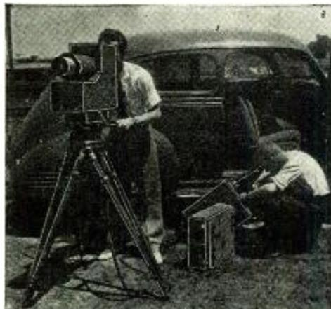
The photos show the new Du Mont television pick-up camera, which is extremely portable and can be quickly set up anywhere, thanks to the specially devised tripod shown in the photo. The necessary amplifiers and other apparatus are arranged in portable cases, and the whole television pick-up camera outfit can be dispatched anywhere on short notice, in an ordinary automobile.
