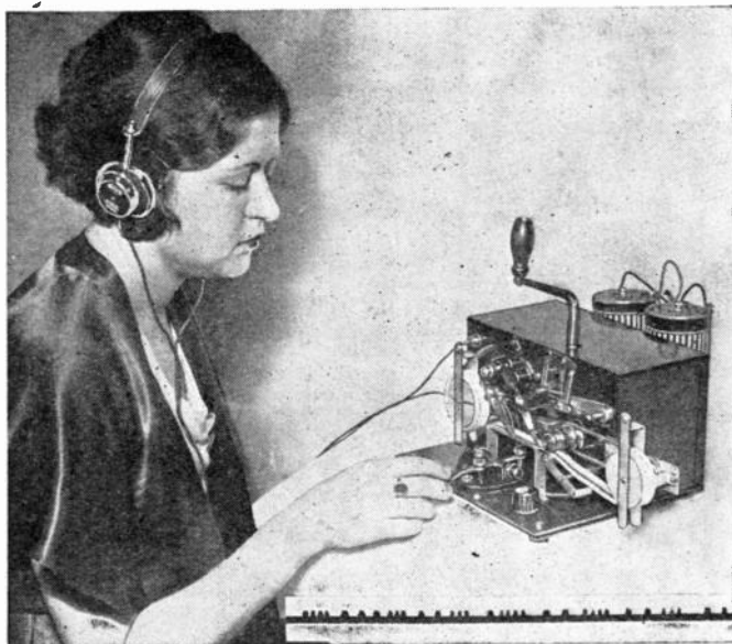
Latest code teaching machine also records your "sending" for comparison. Sample of code record at lower right.
