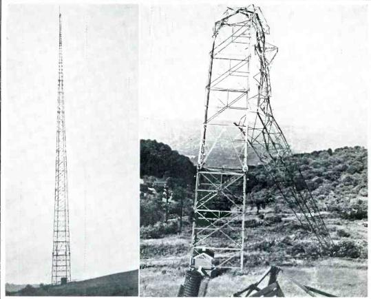
With the increasing number of stations came interference problems and directional amtennas such as this 1940 twin-tower transmitter plant of WCAE, Pittsburgh. In 1944 a tornado crumpled the tower on the left. Station switched to an auxiliary. (WRYT)
