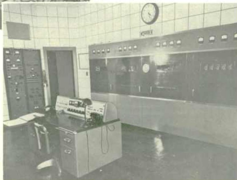
*Here is the inside of the building showing the 5,000 watt transmitter installation.*
