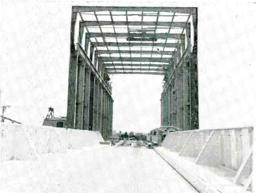
Framework of Garrison Dam intake structure is perched atop huge concrete pillars housing eight power and flood control tunnel gates. The structure is higher than the capitol building in Bismarck. Below, KFVR broadcasts a bid opening on ten million dollar powerhouse. Left to right, news editor Jack Swenson, reporter Stan Wilson, Garrison District Engineer Col. R. J. B. Page and assistant.
