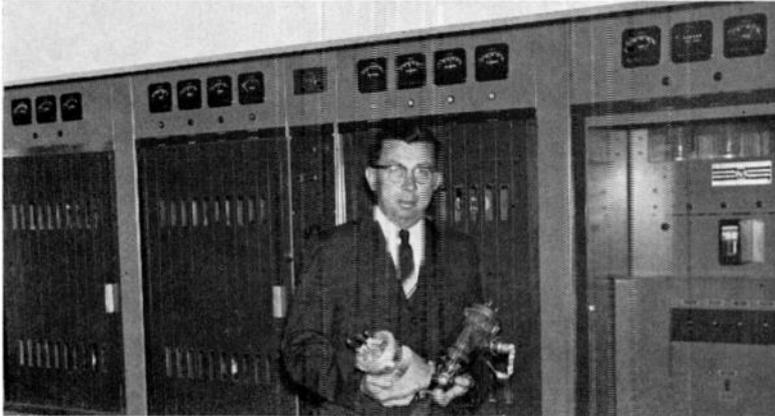
At left, chief engineer Don Burcher in front of the KMA transmitter at the KMA towers, looks over two transmitter tubes. Generating extreme heat, the old, long-necked tube is water-cooled, the new model cooled by forced air.
