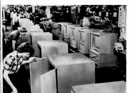
Cabinets undergo final inspection on RCA Victor's TV assembly lines,
