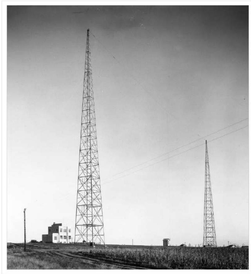
WAAW Towers at 60<sup>th</sup> and Girard Streets. Nearly invisible is the antenna strung between the top of the two towers, it's feed line dropping straight down from the center point to the small building below. (1931) (Courtesy Durham Museum)
