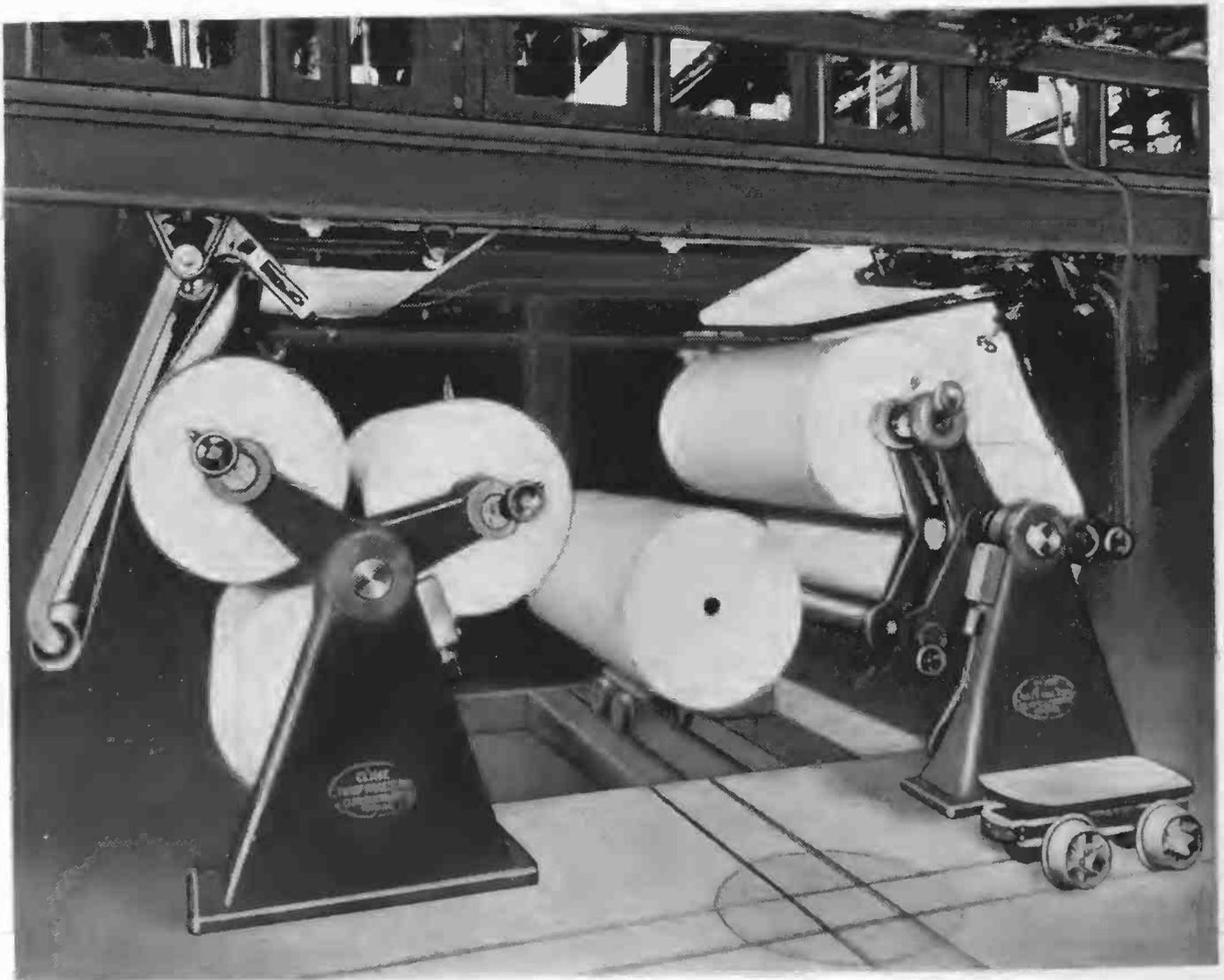
*FROM these reels newsprint feeds from the basement of The Tribune Plant up into the presses. As a roll is exhausted another takes its place without stopping the presses.*
