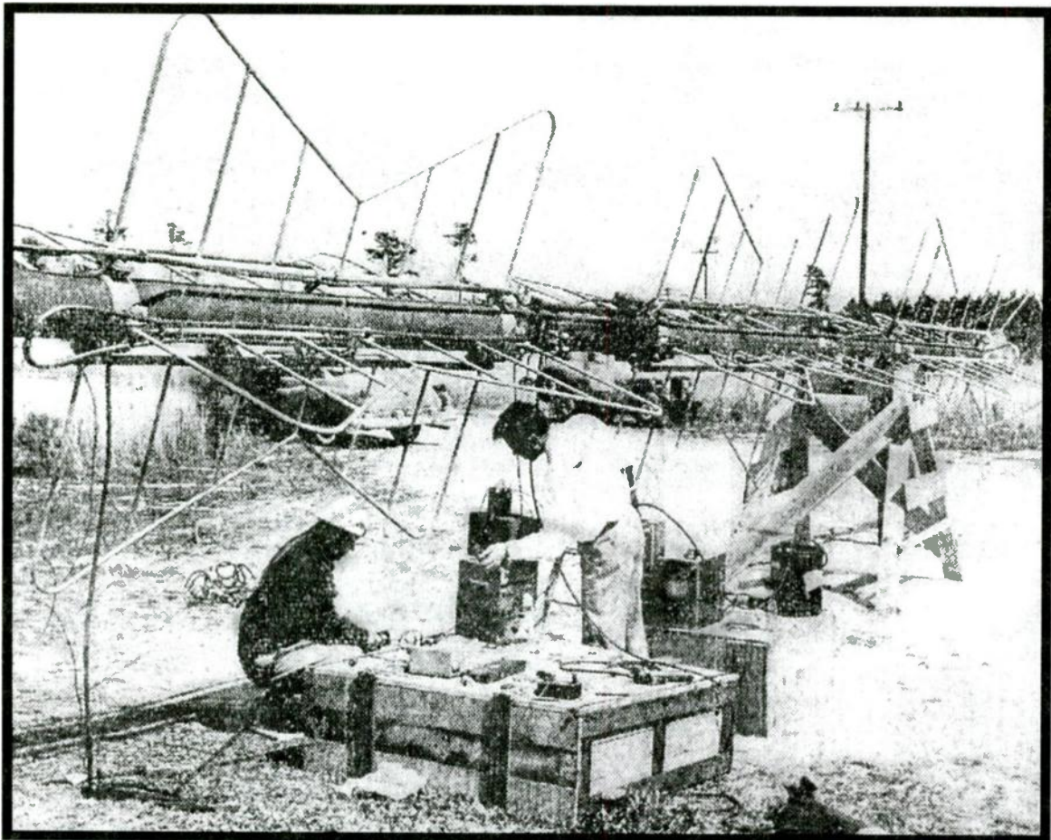
The giant antenna for WMFD-TV’s transmitter, located on the banks of the Cape Fear River near Orton Road, is tuned by technicians before being raised. Regular programs from Wilmington’s first television station began on April 9, 1954. The antenna weighed two and a half tons.
