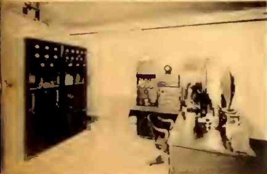
**NEW TRANSMITTER** was erected near Cook Paint factory in North Kansas City, in 1930. A 1,000-watt Western Electric set; licensed to operate daytime only with 500 watts.
