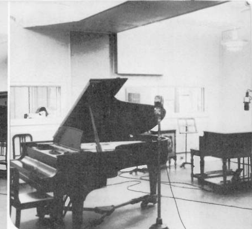
STUDIO C. Hinged panels on wall are for adjusting the studio's acoustics to fit each program.
