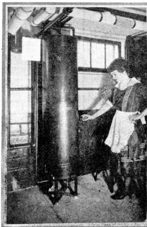
The hot water-back in the kitchen range with its tendencies to explosion is here abolished, and the quiet electric current warms the water for the entire household.
