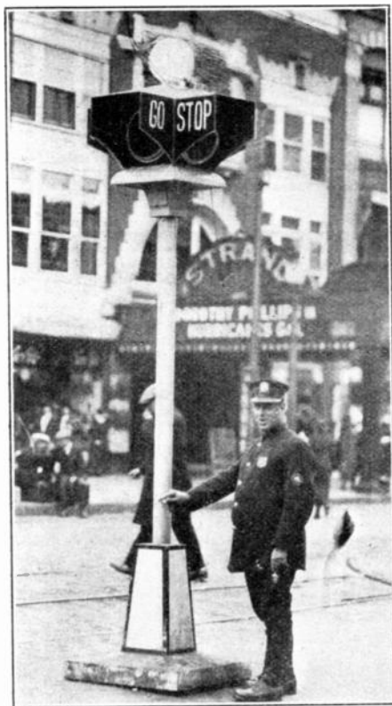
The so-called iron policeman—an improved traffic controlling semaphore, electrically lighted, the color of the lights giving indications in addition to the inscriptions.
