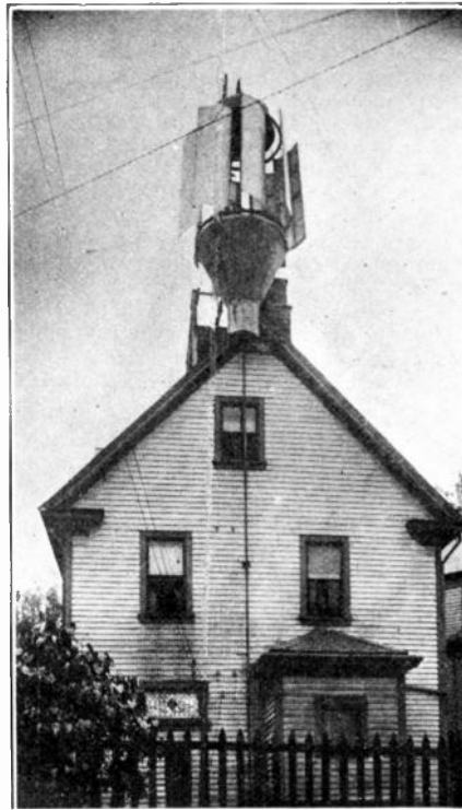
The wind motor on the gable end of a building, a very practical application of it.
