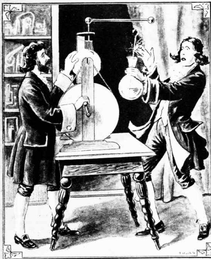
Pieter van Musschenbroek, in the University of Leyden, 1746, connected the water in an insulated glass vessel to a static machine. The vessel showed unexpected electrical activity when it discharged through the body of Cuneus, who attempted to remove the connecting wire from it.
