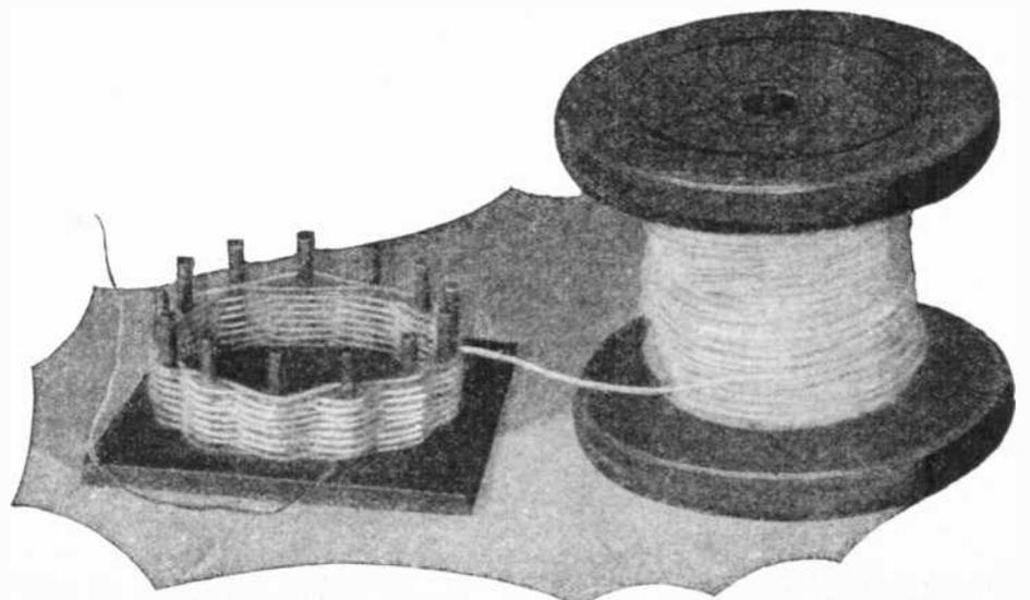
Method of winding the low loss coil—13 pins screwed into a metal base in a circle of three inches in diameter constitute the winding form.
