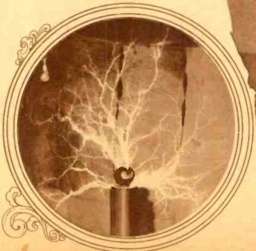
The terminal of the large Tesla coil in full action is shown at left. Some of the sparks are more than eight feet long.
