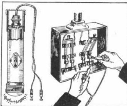
A very ingenious attachment to the ordinary flashlight is illustrated above. It consists of a metallic case which can be screwed on the base of the ordinary flashlight case and which contains a pair of insulated wires connected to the terminals of the battery. The other ends of these wires are brought into contact with the terminals of the circuit to be tested. If the circuit is not "open" the flashlight will light up.
