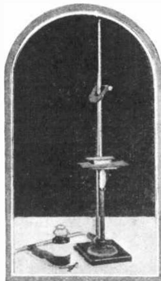
The apparatus for applying the selenium is shown above. A mica or slate sheet is wound with wire, forming a lattice on which the selenium is retained. The mica is placed on an iron plate in an aperture wherein the bulb of a thermometer is set, and the plate is heated until the selenium spread on it melts, careful regard being given to the temperature.
