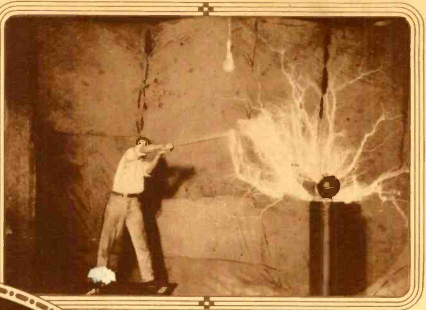
The torch bearer below stands in a basin of salt water connected to the Tesla coil. The torch is a strand of wire from which powerful sparks shoot into the air.
