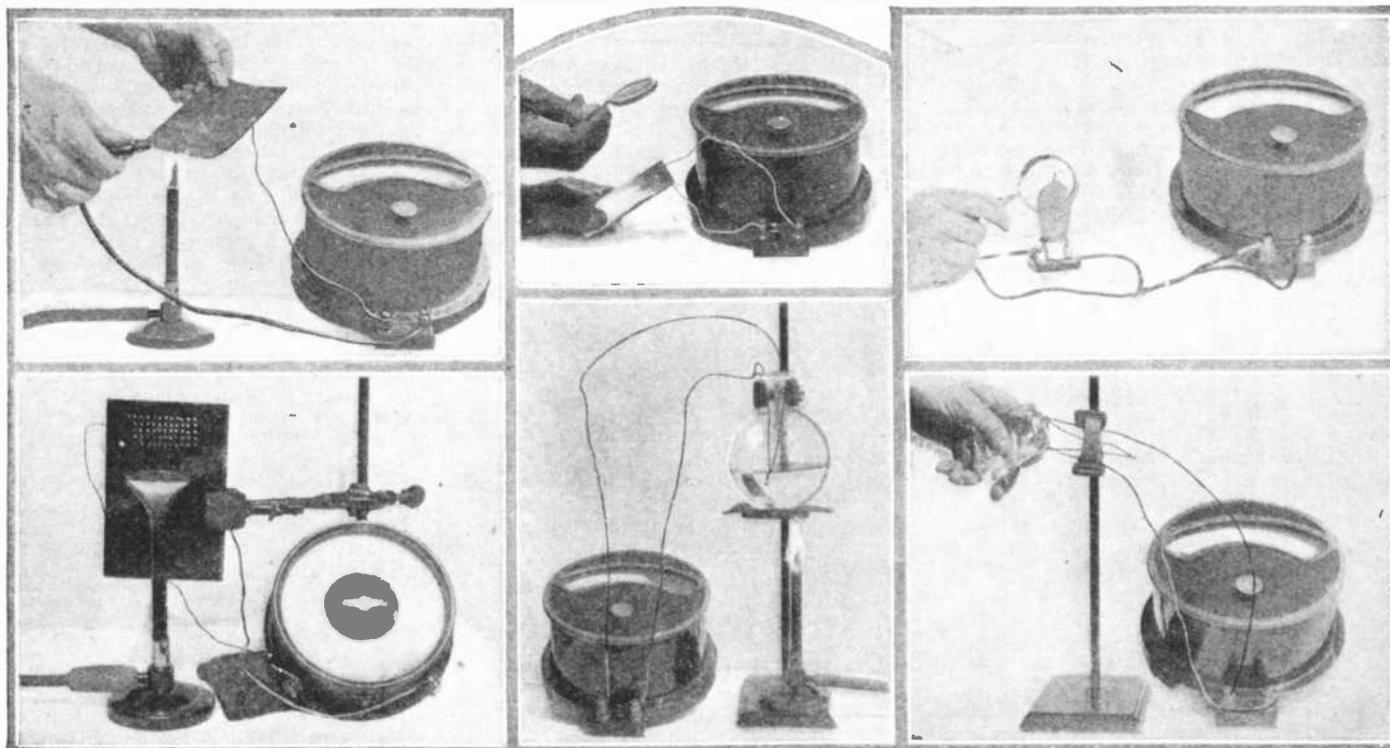
The thermo couple is an endless source of experiment. Some can be made sensitive enough to detect the heat due to solar rays focused on them by a weak lens. They can be used to give the temperature of heated solutions and a number of them connected in series will form a battery of considerable potential. Such a battery is shown at the lower left. The couple is as sensitive to cold as to heat, as illustrated in the picture on the right.
