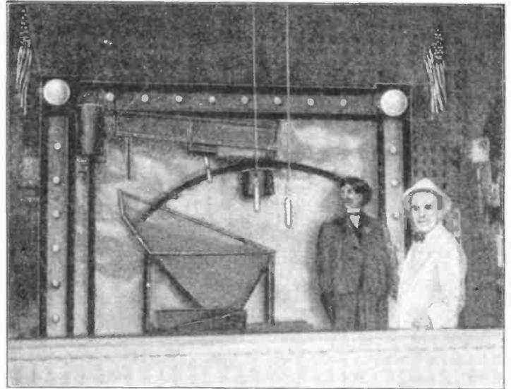
The "Candy Kid" accomplishes the selection of one out of a number of balls. A silk hat automatically removed from the head of the figure receives a number of balls and tips them into the hopper where one of these is lodged in a cavity and the rest roll by into a small cart. The retained ball carries the lucky number.
