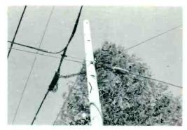
AND AFTER! Twin lead gone. Fower transformer gone. Line amplifier boxes gone! But, same pole. Now all line amplifiers mount at the base of the poles, and 110 volts is "on the ground" as prescribed by law. Coax feeds the system, in place of the seven-year-old flat line.
