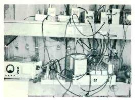
HEAD END—600 feet above Mariposa, 2,600 feet msl, Perry's head end shack cranks out the microvolts 24 hours a day. Channels 4 and 5 from San Francisco are fed into Jerrold 406A Amplifiers, and then into a Jerrold DPM unit. Channels 24 and 47 Fresno, are converted in old MA4-1 units (Blonder Tongue) which will be replaced by new MUC converters now on order.
