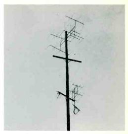
"TOP OF THE HEAD END"—60 feet above the top of Perry's television hill, yagis for VHF and corner reflectors for UHF scoop up the microvolts to feed the system. San Francisco is 120 airline miles, Fresno UHF transmitters "line of sight" over a 30 mile path.
