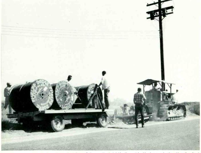
Antennavision construction crew making underground installation of Aluminum Sheathed Cable. The special cable plow precedes the cable trailer, directly behind the Caterpillar tractor, automatically filling the trench with cable. A grader follows to fill in the trench.
