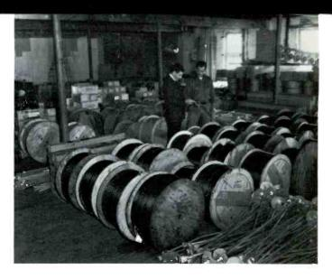
Mauntoins of electronic equipment, including 378 miles of cooxial cable, 150 miles of strand support wire and 236 amplifiers filled a Wilmington warehouse in November of 1961.
