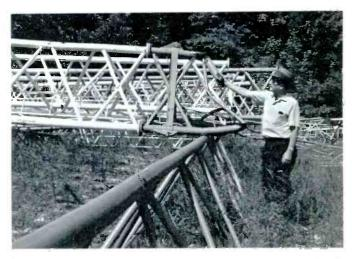
Stacked pieces of damaged tower. Cut guy wire was responsible for damage shown here.
