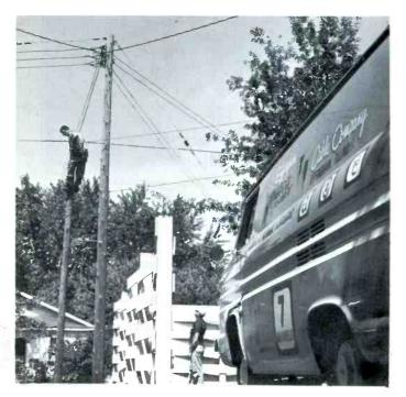
System technician making hook-up at top of company pole. Adjacent pole is owned by local utility company.
