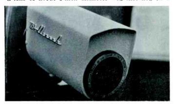
Equipping a camera with a remote pan and tilt unit and electrically controlled Zoom lens allows one-operator operation.
