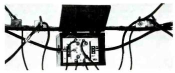
THE 36 INCH CORR-O-FOAM enters a multi-taps outlet and four RG-59 house drops carry the signal directly to the subscriber's sets.
