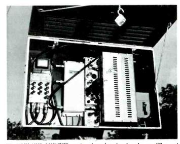
SKL MAIN LINE AMPLIFIER receives incoming signal and reamplifies and retransmits it to the main trunk line along % inch Corr-O-Foam to the next amplifier station.
