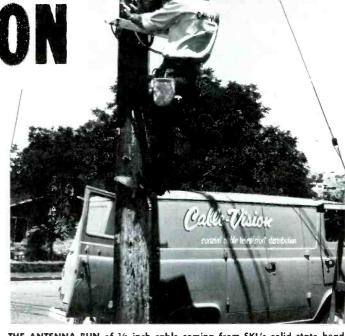
THE ANTENNA RUN of 1/2 inch cable coming from SKL's solid state headend amplifier is adjusted by Cable-Vision technician.
