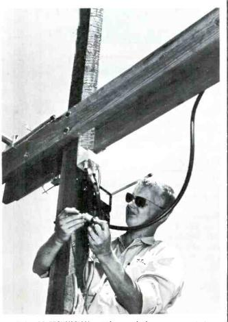
CLOSE-UP OF TECHNICIAN, running continuity test on 1/2 inch 75 hm Corr-O-Foam cable.
