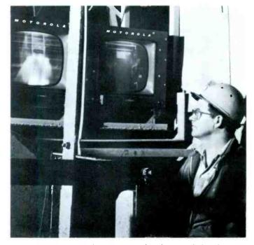
Hoist operator at the Southwest mine watches dumping of skips by means of closed-circuit television system.
