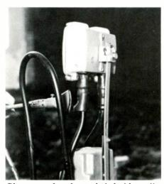
Close-up of a heat-shrinkable splice cover in action. Flame spreader produces even heat, making flame invisible.
