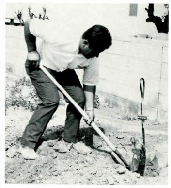
New style pedestals used in Yuma system are knifed into loosened earth. Sandy soil in that area makes installation operations even easier.
