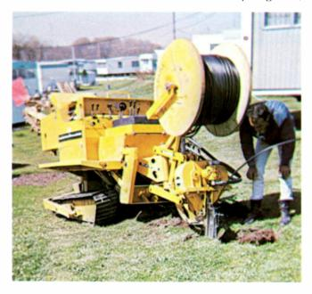
Start of direct burial run, with vibratory plow in ground, is shown here. The method eliminates trenching, hand laying of cable, and backfiling.
