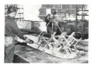
FINISHES Hot-dipped galvanizing after fabrication
