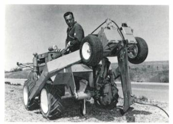
Optional plow attachment quickly converts 30-horsepower trencher to vibratory plow for direct burial of cable. This trencher model provides trenches of up to 18 inches wide, 6 feet deep, and is equipped with hydraulic backfill blade. Additional attachments convert basic trencher into backhoe or boring unit. Will handle all sizes of distribution cable.
