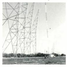
high gain and directivity to furnish interferencefree reception. Features space diversity — use of two antennas connected by an automatic switching unit sampling response of two antennas. If fade is experienced on one antenna, head-end equipment is switched to the alternate to provide the best possible picture available at all times.
